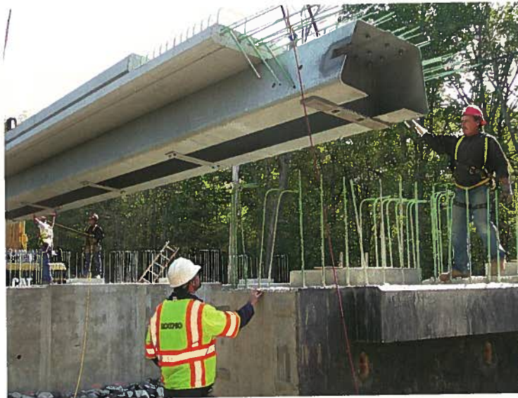
Photo 2: Erection of a prefabricated superstructure module.
