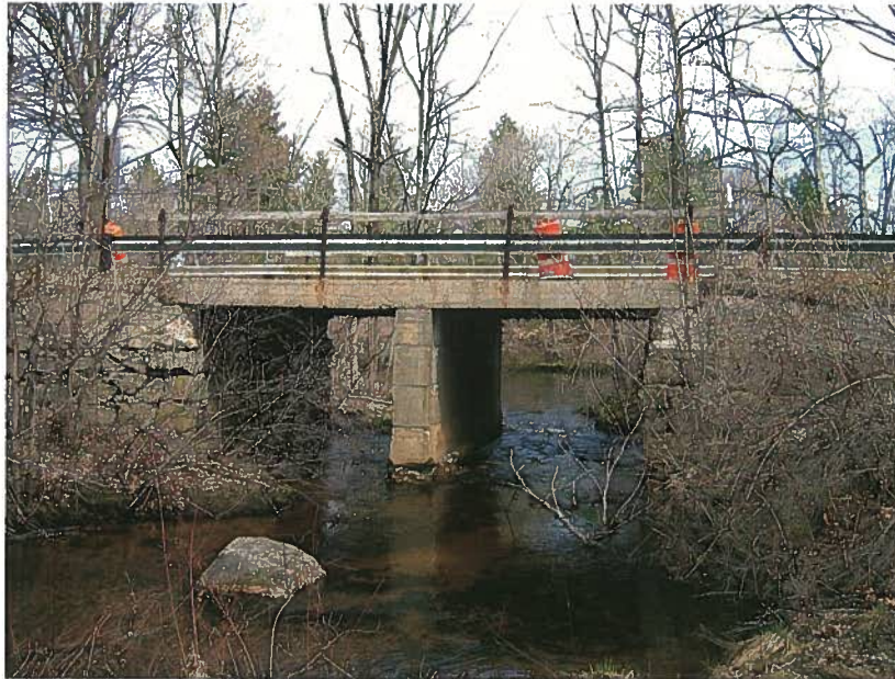
Photo 1: Former bridge supporting River Road over Ironstone Brook.
